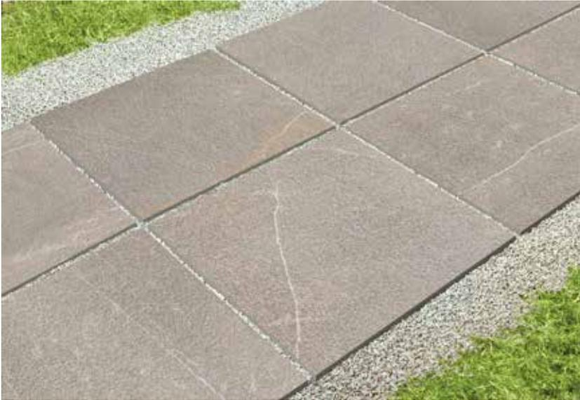
This system is particularly recommended in areas where drainage of the water in the underlying soil is a problem, and also for concrete floor screeds, such as on balconies or terraces. The slabs can be dry laid by simply placing them on top of the previously prepared gravel base, without the need of porcelain stoneware adhesives. This means the slabs are easily levelled out on top of the gravel and are ready for use immediately afterwards.
