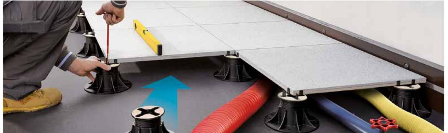
Floating paving is composed by a series of modular and adjustable supports, that easily and safely adapt to all paving types. Designed to guarantee an homogeneous surface, without bringing radical changes to the existing structure, as well as to eliminate humidity problems, water infiltrations, passage of electric cables and pipes, floating paving solutions allow easy and quick inspections and rainwater efficient drainage.
