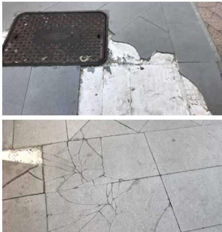
Paving with increased thickness to 2 cm guarantees high mechanical and resilience (ability to absorb shocks) properties, to avoid any breakages due to the inability to take heavy loads, such as vehicle crossing and stresses caused by temperatures below zero. These inability is typical for pavings with lower thickness. Therefore, L'Altra Pietra is the perfect paving for many different uses in outdoor environments.
